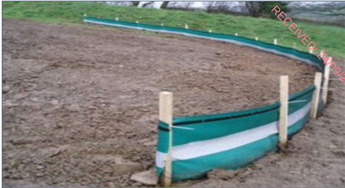
Plate 3-4 Embedded Silt Fence
