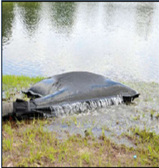
Plate 3-1 Silt Bag with water being pumped through.
