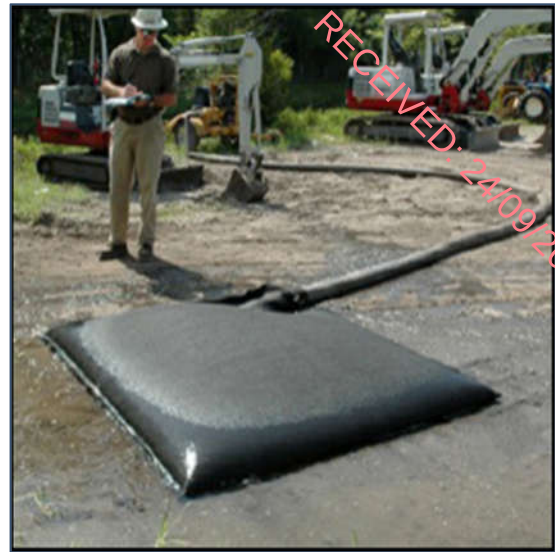
Plate 3-2 Silt Bag under inspection
